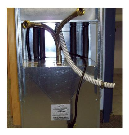
The hoses and electrical cord shipped already attached to the chassis. Refrigeration Chassis and ERV installed in cabinet equipped with a hinged door.
