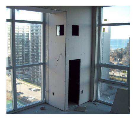
Drywall installed and the cabinet remains empty of any refrigeration or electrical components throughout the construction site period.
