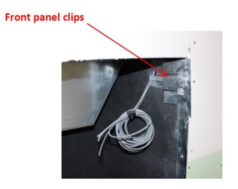
The thermostat wires are brought into the cabinet. The front panel clips are installed in the cabinet.
