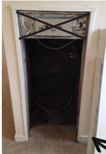
Chassis gets installed into existing cabinets
