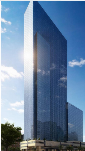
MIMA, W42ND ST. LEED GOLD NYC, NY 1700 BULLDOGS
