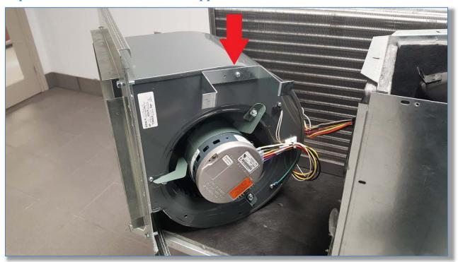
Step 6: Using the self-drilling screws, remount the hat bracket on the opposite side of the Blower.
